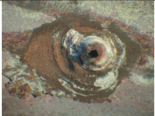
Fig. 10b – Case 7 Type 1 pitting – close up of pit
