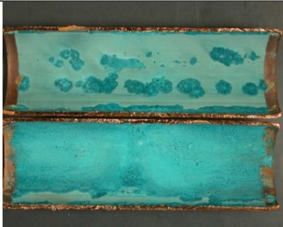
Fig. 12a – Case 8 Type 1 pitting -bore before cleaning
